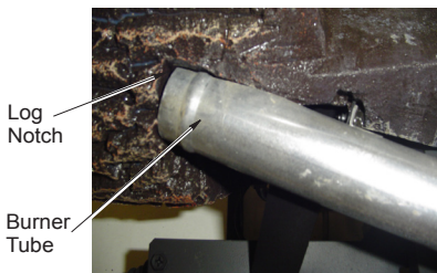
Figure 29A - Installing Back Left Log
