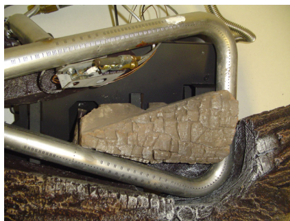
Figure 27A - Installing Charred Log Top View
