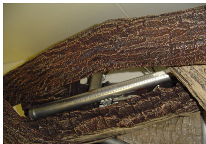
Figure 31A - Installing Back Top Log, Top View
