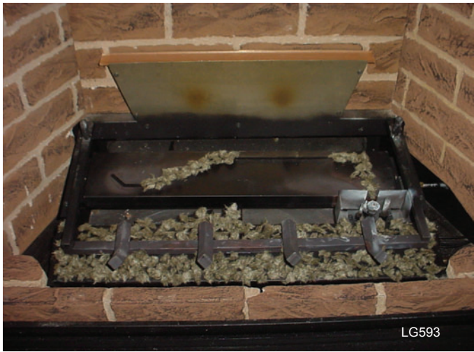
Burner Grate Assembly
